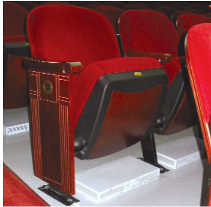
Typical floor-level diffuser from floor level (left) and below (right).
